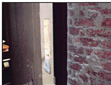
Using the hole saw, I started cutting out the cavity for the mortise lock.
